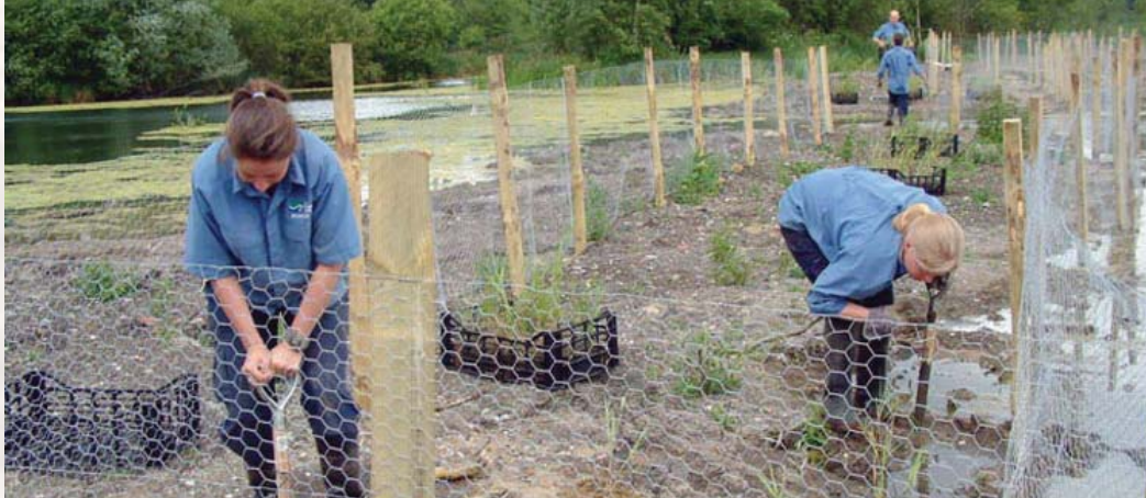
Newly planted reedbeds can also be protected from their biggest threat, grazing waterfowl (especially Canada geese) by using suitable fencing.
